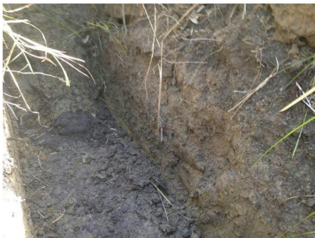
TP5 showing 0.1m of topsoil over 0.6m of alluvial silty clay
